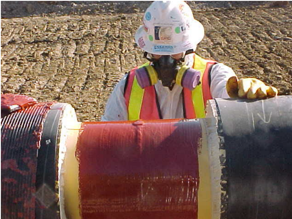
Figure 5. Girth weld coating using high temperature epoxy
